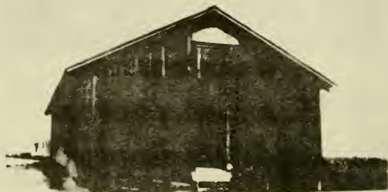
3. A bunk house in an asparagus camp in Sacramento County occupied by twelve Filipino asparagus cutters. This camp is rated "bad" by the Division of Housing and Sanitation.
